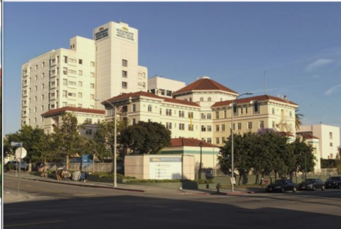
Hollywood Presbyterian Medical Center has shut down much of its network for the past week because of ransomware, causing the diversion of some emergency patients to other hospitals, according to sources at the hospital.
